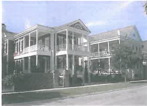
Mount Pleasant, SC The front and side porches of 1 On add interest to a residential street
